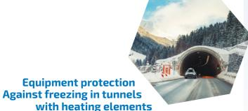
As for the Channel Tunnel, the flexible heating elements are used to maintain temperature of the fire safety equipment or water supply equipment over very long lengths.
